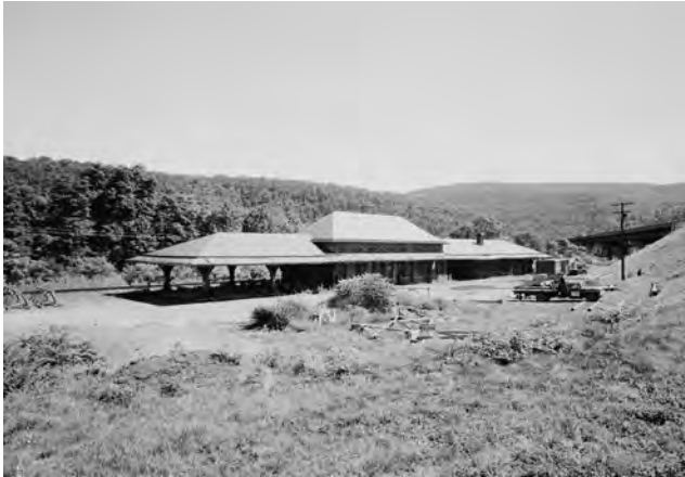
Delaware Water Gap Railroad Station (photo from the Library of Congress )
