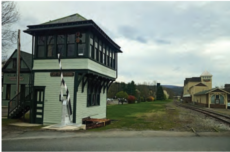
Railroad Switching Tower, East Stroudsburg
